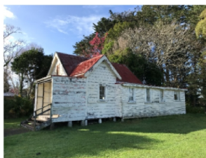
Typical view of the right hand side elevation
